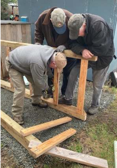
Building the platform
