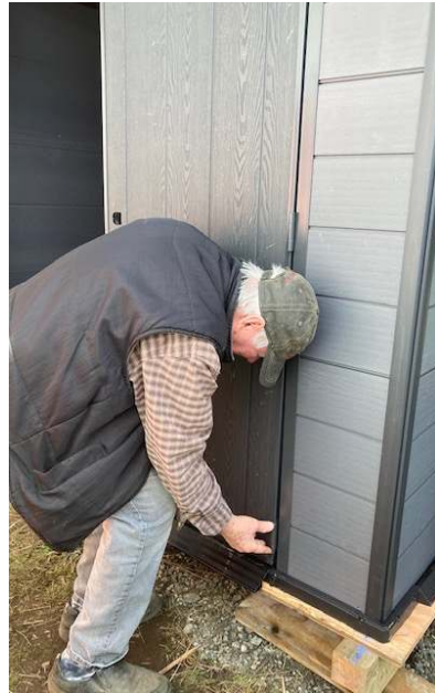
Hanging the doors
