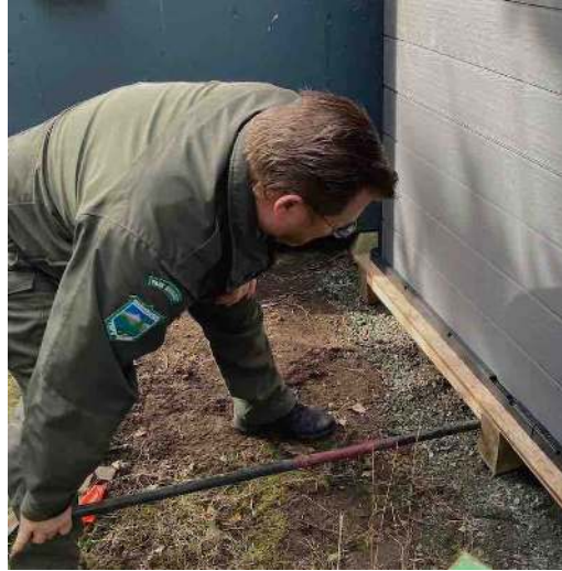
The Park Manager helped move the shed into place
