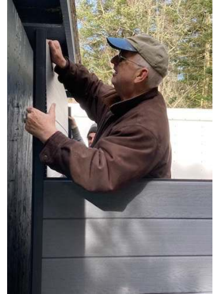
Erecting the sides
